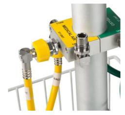
17. Attach the 3-foot oxygen hose labeled **VT UNIT** to the corresponding connection port on the oxygen manifold also labeled **VT UNIT**.
